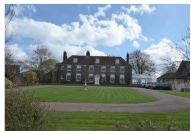
Principal south elevation fo the Dunton Hills farmhouse
